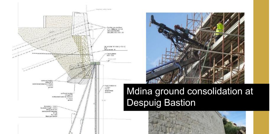
Works on Despuig Bastion involved the pinning of the ground below the ramparts with various rows of large and small diameter piles of reinforced concrete inserted to a deep level into the ground.
